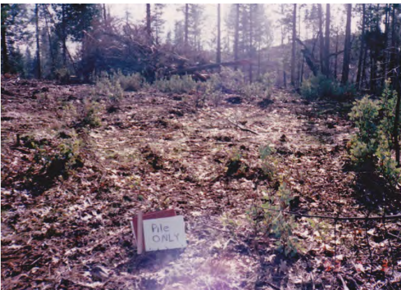
C - Dozer piling only
