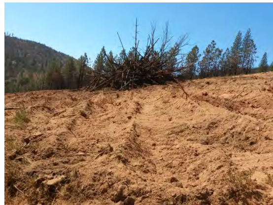
D - Dozer piling, followed by DTFC
