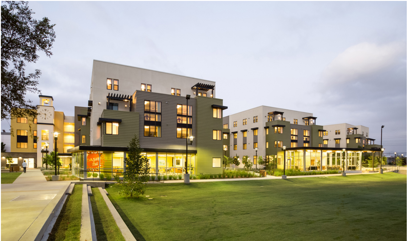
Cabrillo Gateway revitalized a former military base to provide new housing for homeless veterans and families.
