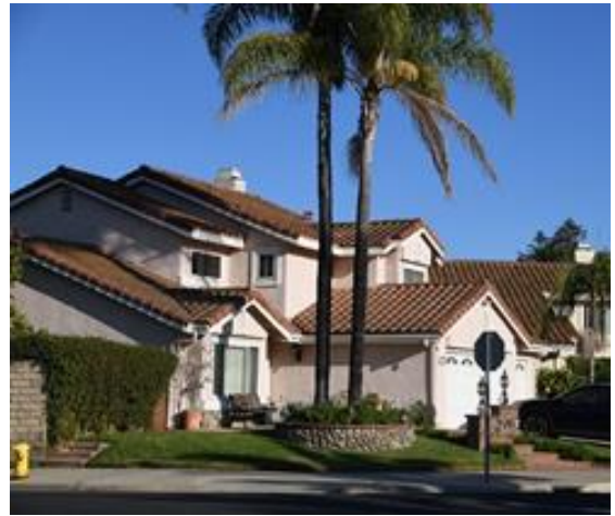
Residential neighborhood in Moorpark.
