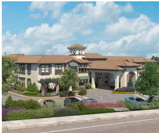
Oakmont Assisted Living, under construction.
