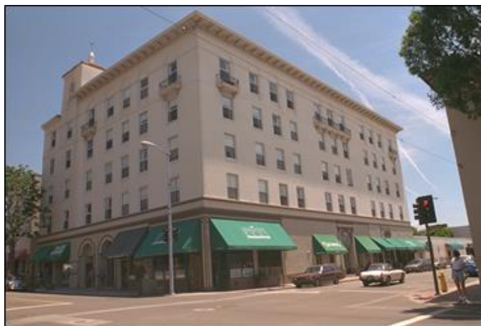
Anderson Hotel, located at the east corner of Morro and Monterey Streets Source: Community Development Department, 2014
