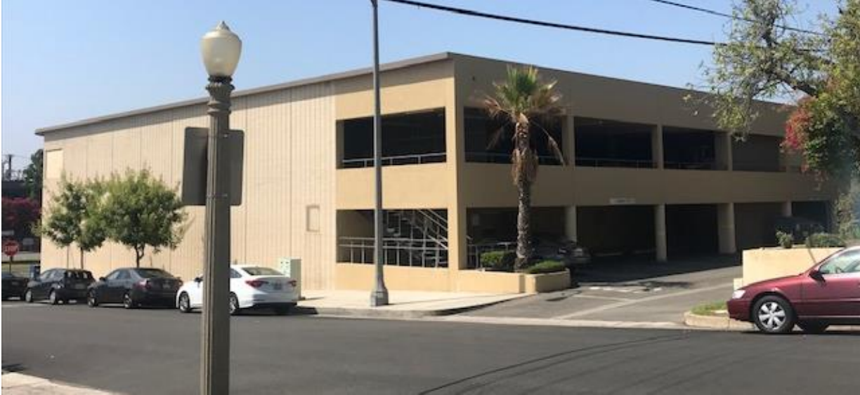
Figure 10: Parking for Wells Fargo Building, 2375 Huntington Dr
