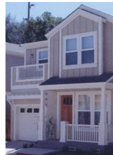
Manufactured Multifamily Home Courtesy of CMHI
