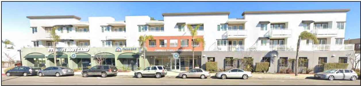
Cabrillo Family Apartments, a 44-unit, 100% affordable development in Downtown Torrance
