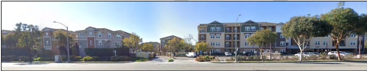
Mixed Townhouse/Senior Stacked Flat (Podium) Development in the Hawthorne Boulevard Corridor Specific Plan, Del Amo Sub-District 1
