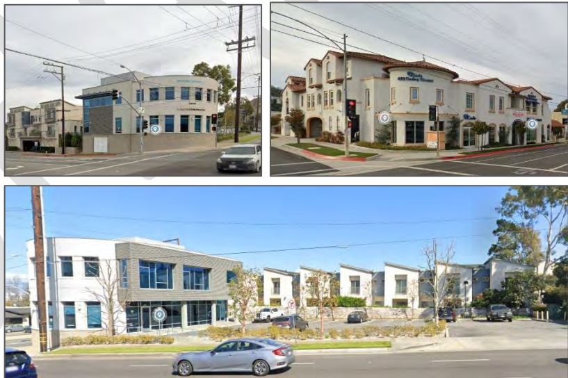
Examples of new mixed-use developments in the Walteria District in the HBCSP
