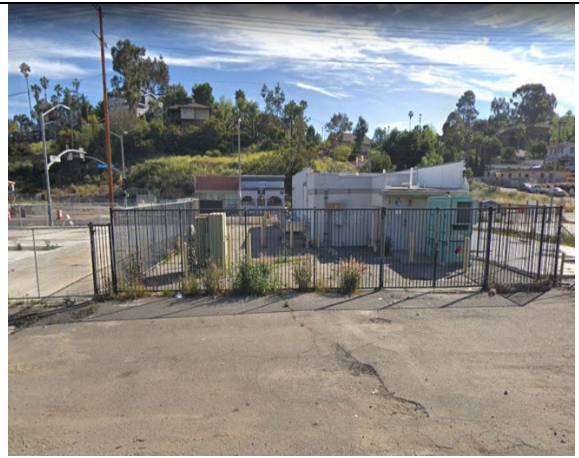
Looking Northeast from Mercantile Street
