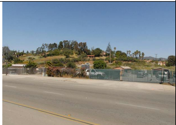
Materials yard consisting of small buildings, shade structures, and open yard storage (viewed from S. Santa Fe Avenue looking east)
