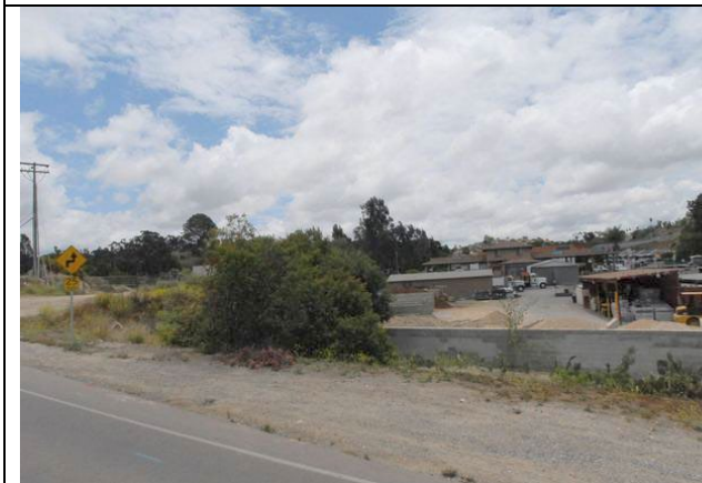
Materials yard consisting of small buildings, shade structures, and open yard storage (viewed from Monte Vista Drive looking south)
