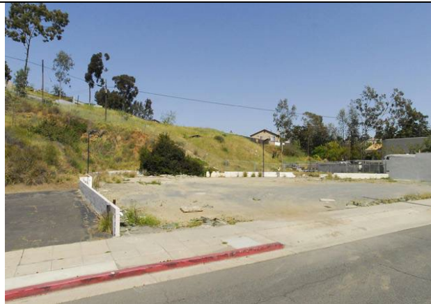
Typical underdeveloped site that had been paved at some point (viewed from S. Santa Fe Avenue looking towards the east)
