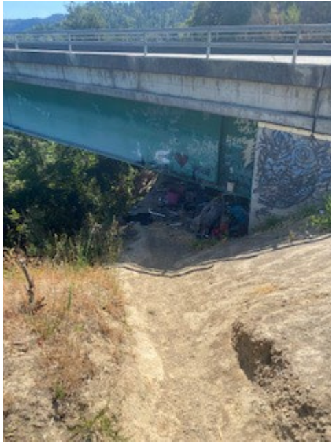
North Bear Canyon Bridge Encampment on ROW
