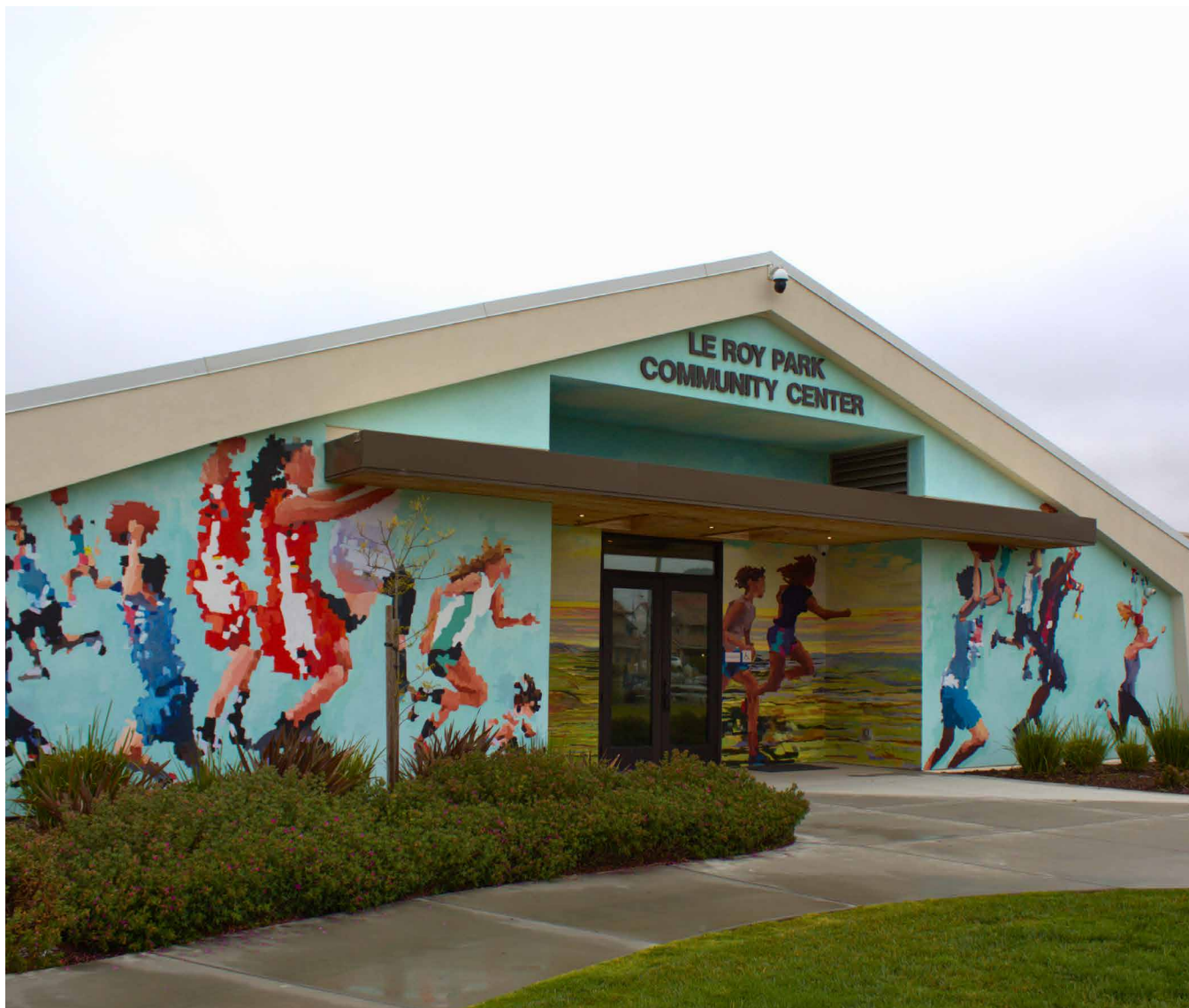
City of Guadalupe Le Roy Park Community Center, Photo Credit: Dayanira Cruz
