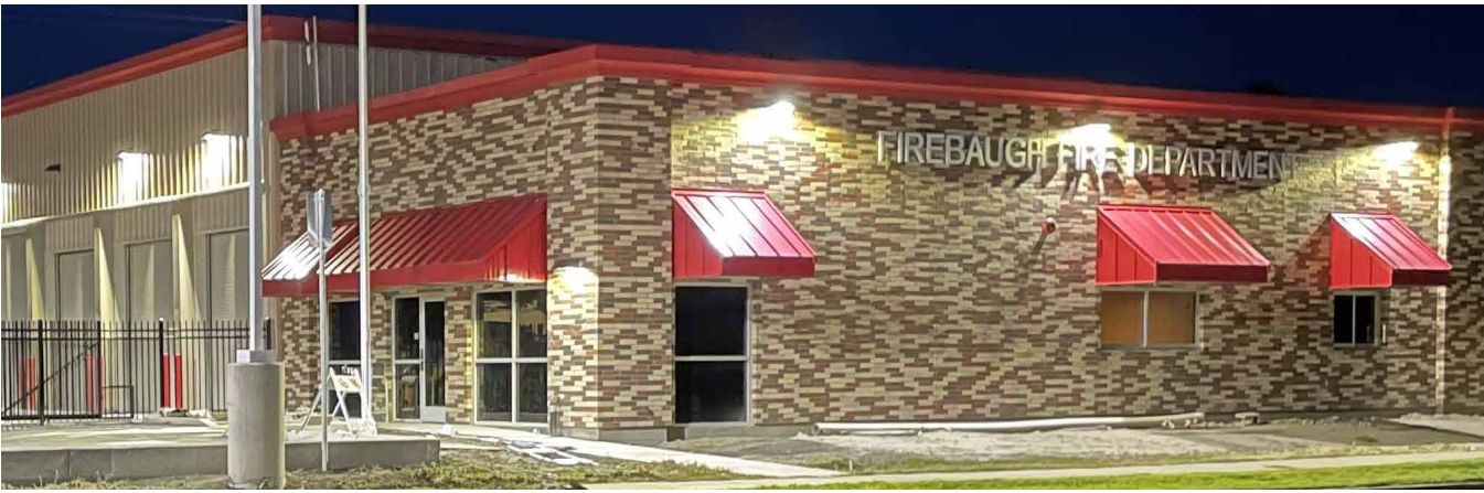
City of Firebaugh Firestation, Photo Credit: Paul Ashby
