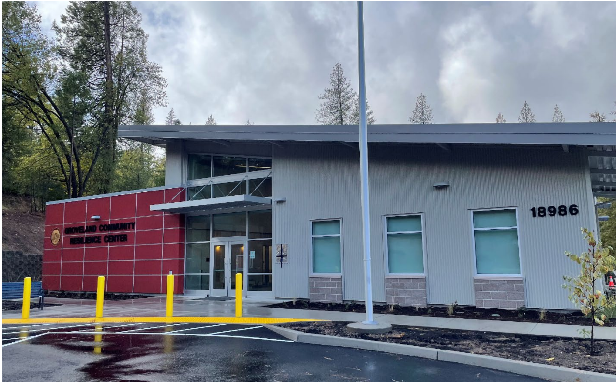
Figure 2: Exterior photograph of Groveland CRC
