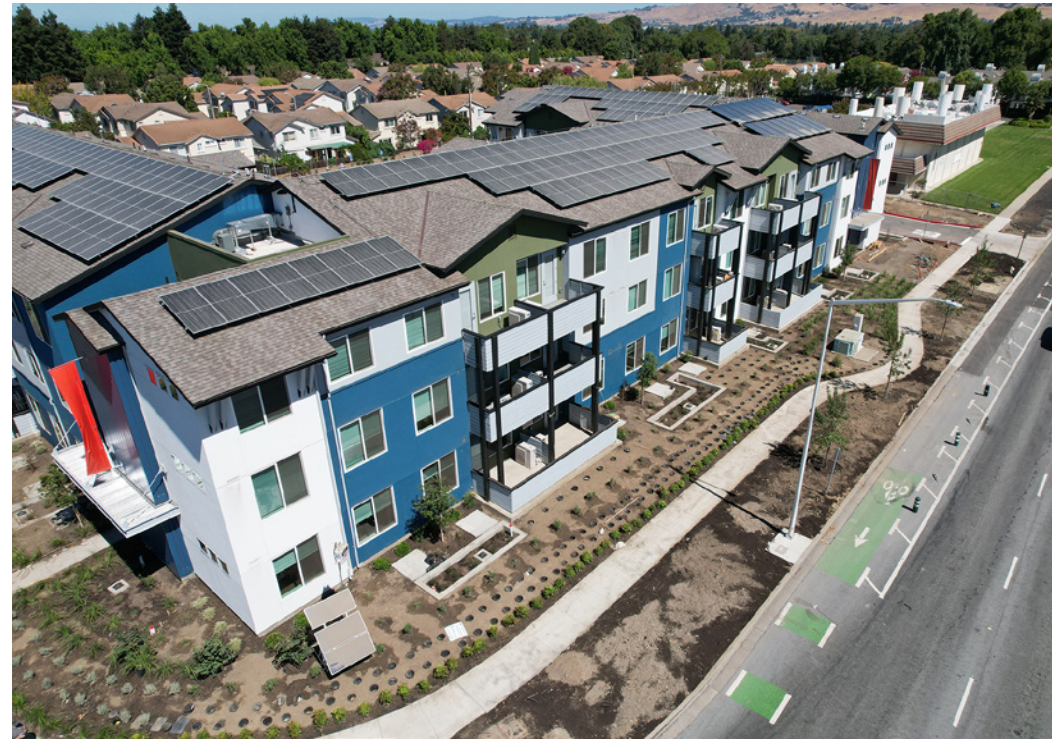
The Fremont Family Apartments, located in Fremont, CA, has 54 units comprised of one, two, and three bedroom apartment homes. The community will provide permanent supportive housing for homeless individuals and families, as well as other affordable units. It includes 26 units for NPLH-assisted tenants. Photo courtesy of Abode Services.
